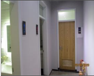
Photo of the sanitary facilities 133 Toilet.JPG
