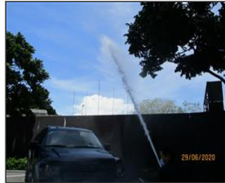
Photo of fire safety equipment 43 Water pressure testing.JPG
